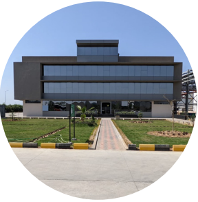
Dahej Facility (I)
