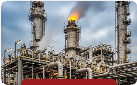
Tail gas clean up for sulphur recovery units
