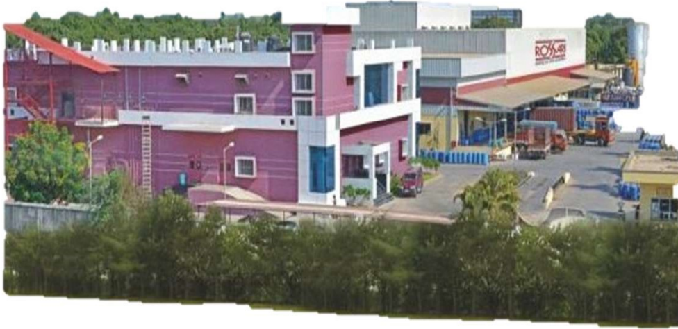
Existing Plant - Silvassa
